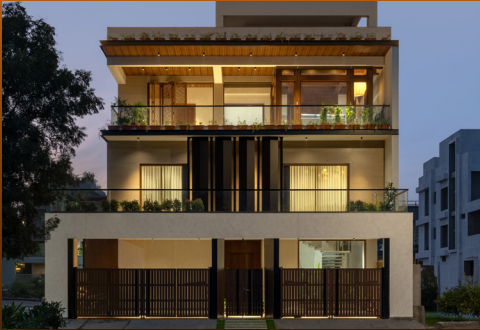
AUR Between Voids
